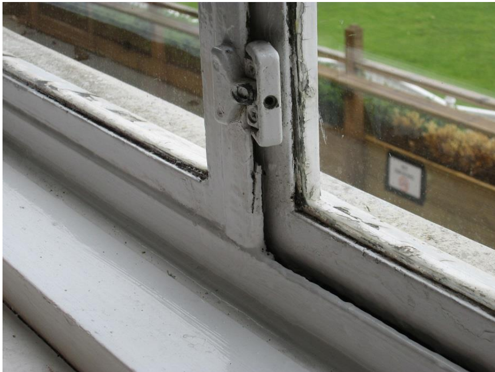
Figure 5.4 Metal window frames with gaps, bar area.
