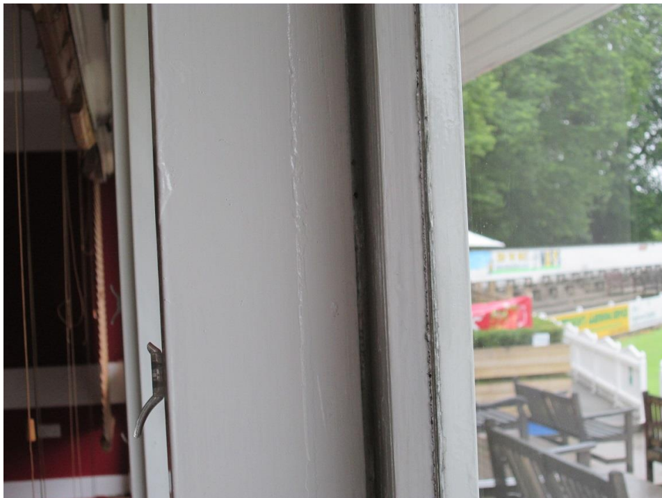
Figures 5.2 and 5.3 Sliding door in Pavilion Suite showing excessive air gap and ground level glazing detail
